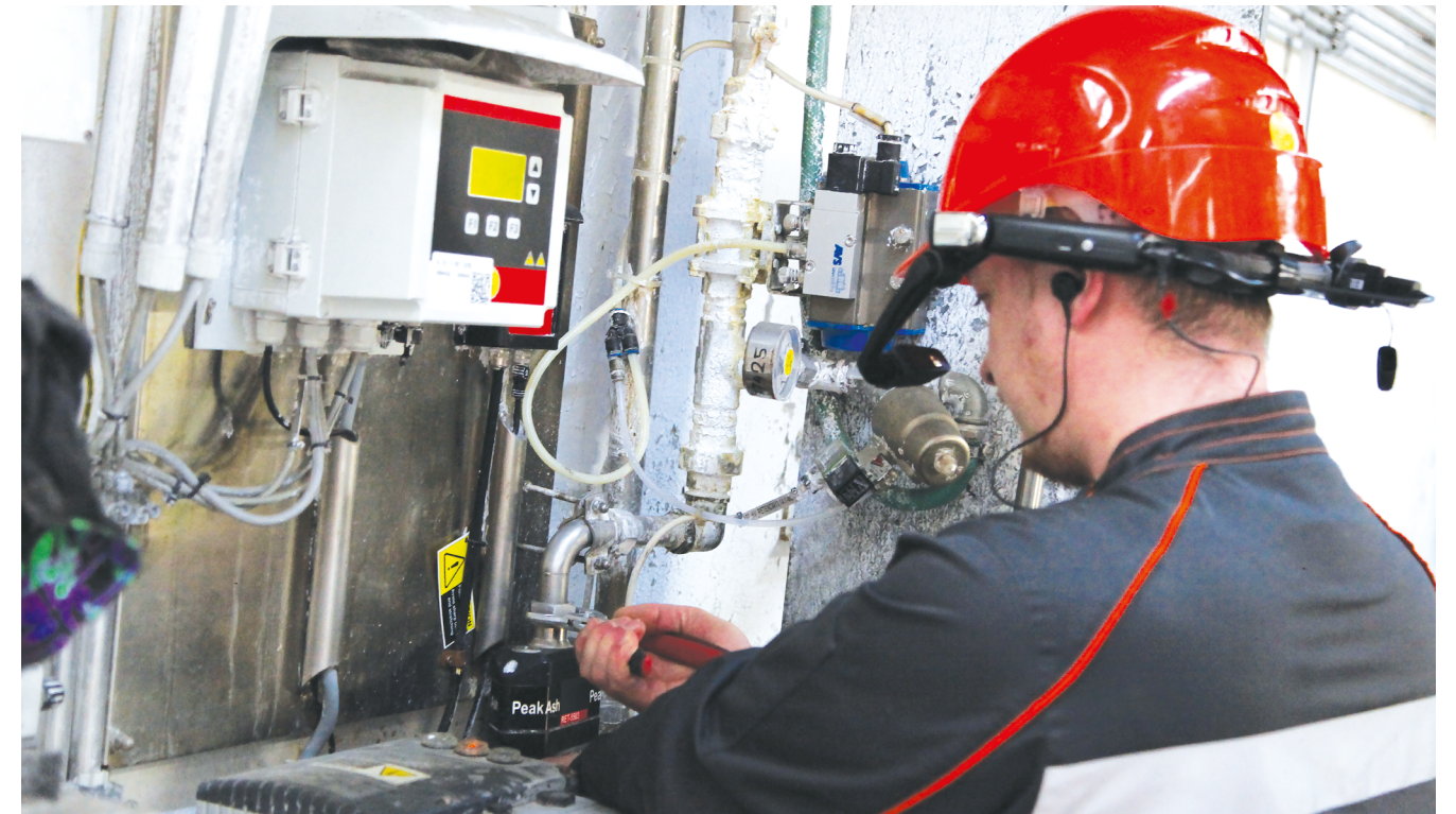
Service and maintenance technicians have both hands free to work all the time.
